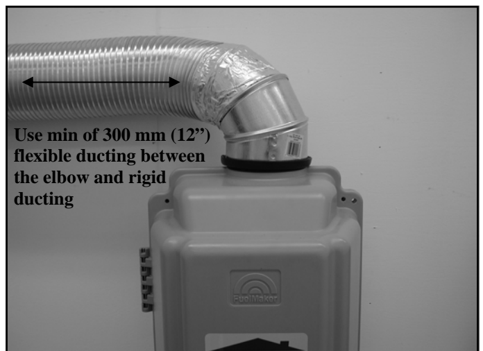
Figure 16 Mating duct to Top Vent Coupler
